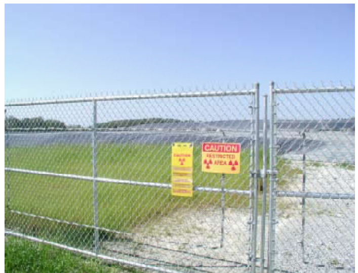
Interim cover for the Maxey Flats low level radioactive waste site in KY.
